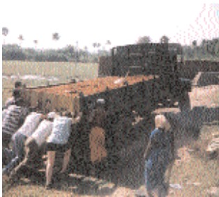
Working with IIFWP, this service project in India saw 30 young people from different backgrounds build the foundations for an interfaith children's home.
